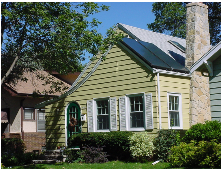
This north Minneapolis home has both a solar photovoltaic (electrical) and a solar thermal (hot water) system that meets about 25 percent of its residents' energy needs.
